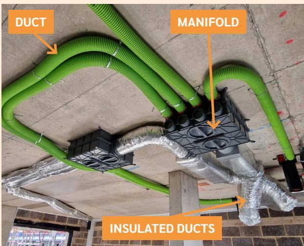
**4 Ensure airtight, secure duct connections to prevent leakage.**
