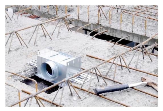
4) Visually check to ensure all ductwork is secured in place, no damage, all gasket seals have been installed and all grille housings are aligned.
