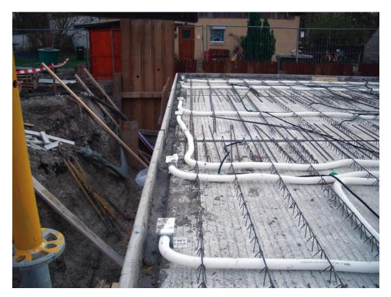
5) Underside of Slab showing 2 x 10 port manifolds awaiting final connection of comfowell silencer/manifold. For Vireo, this will be a 6 port manifold.
